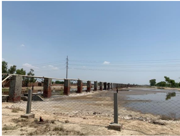
Figure 13: Settling ponds at the CEPTP
